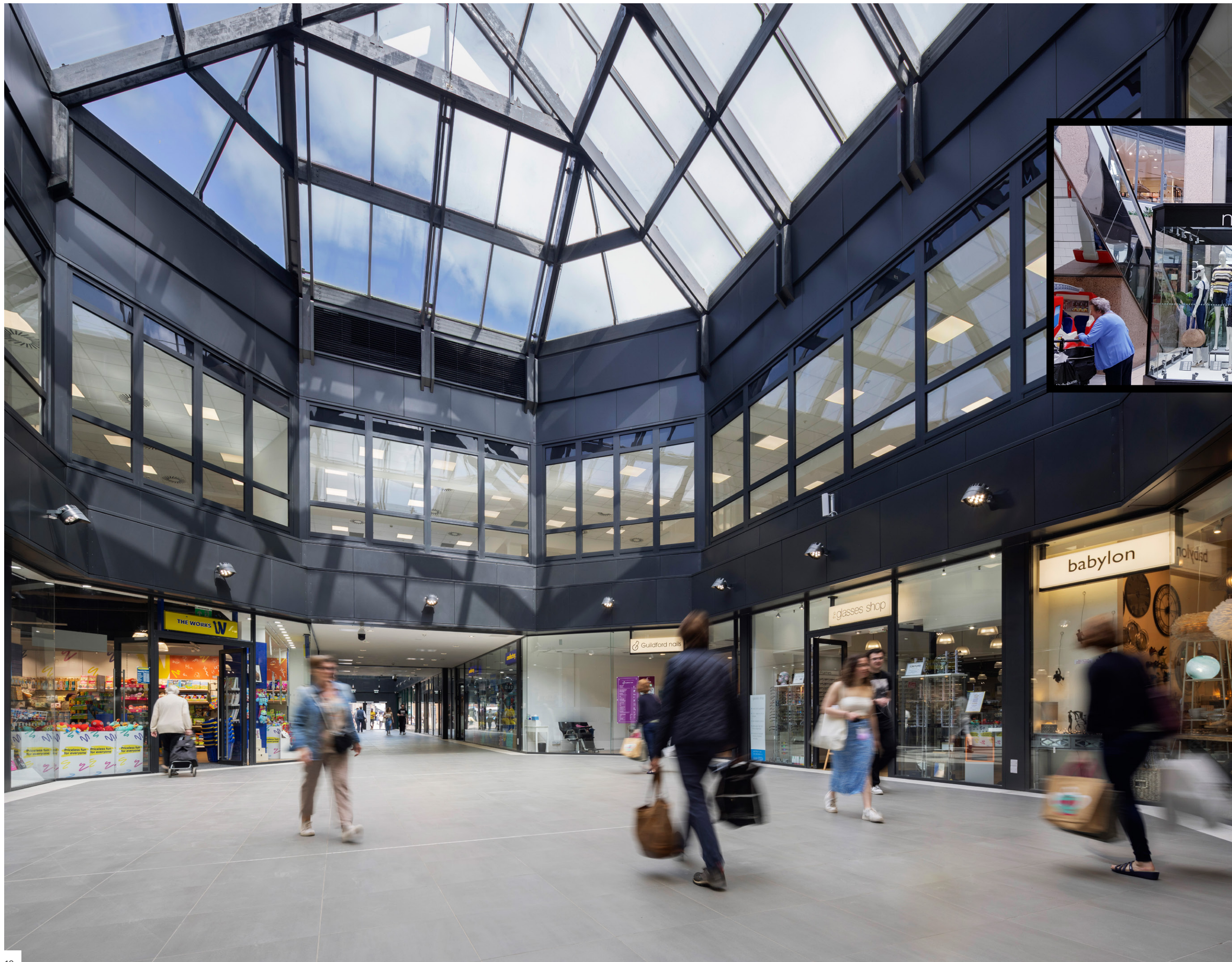
Before & After: New central atrium with lifts and escalators removed and new glazing to first floor
