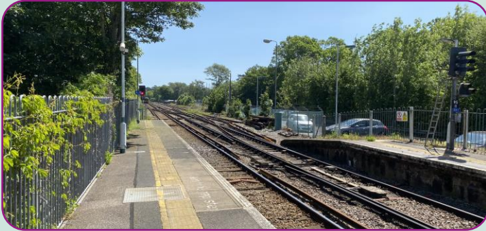
Reigate station - view of the DC rail, 2023 (NR)
